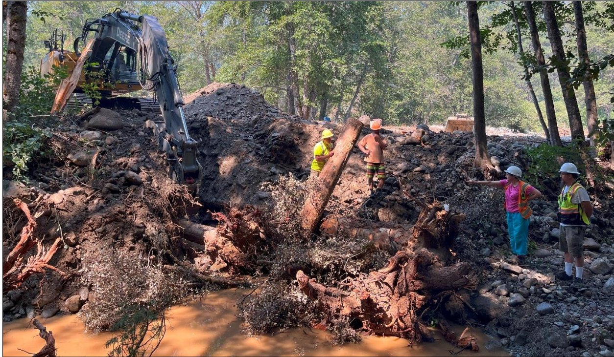
Image 7 (above): Constructing/restoring the Lower Primary Side Channel. August 2023.
