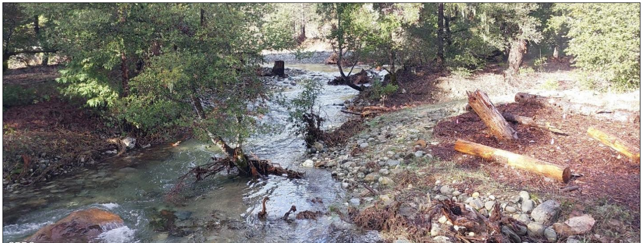
Image 17 (above): Improvements to connection between Far Side Channel and Primary Side Channel (upper Far Side Channel) were made in phase two of implementation. Photo from December 2024.
