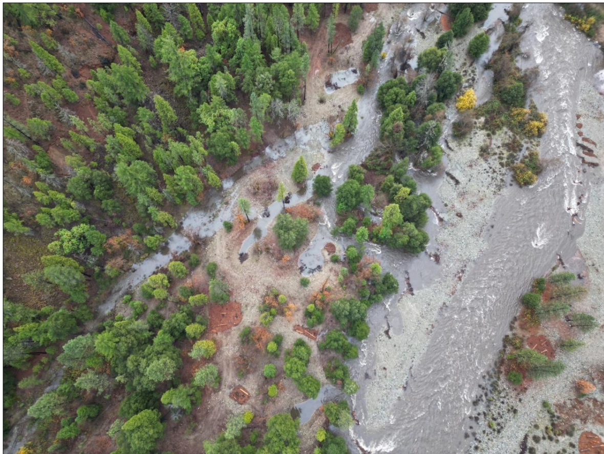
Image 8: High flows on November 22 nd , 2024 fully engaged project features and provided velocity refugia throughout the site. Aerial photo of the Primary Side Channel (on right) and the Far Side Channel (center) with Backwaters 4, 5, 6, 7, and 8 visible at approximately 20,900 CFS at the Salmon River gage on its descent after a peak of 21,700 CFS.
