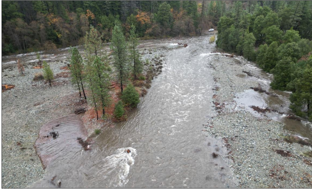
Image 15 (above): Primary Side Channel activated in the first high flow event post-phase two (facing upstream). Photo from November 22 nd , 2024 as the hydrograph was ascending, at approximately 20,900 CFS (at the USGS gage).
