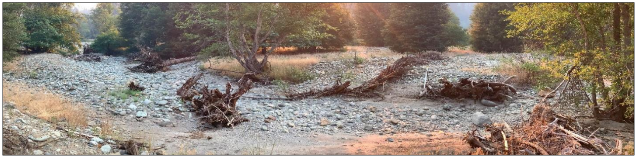
Image 20 (above): Far Side Channel post-phase one implementation, July 2024. This segment of far side channel work was completed in phase one.
