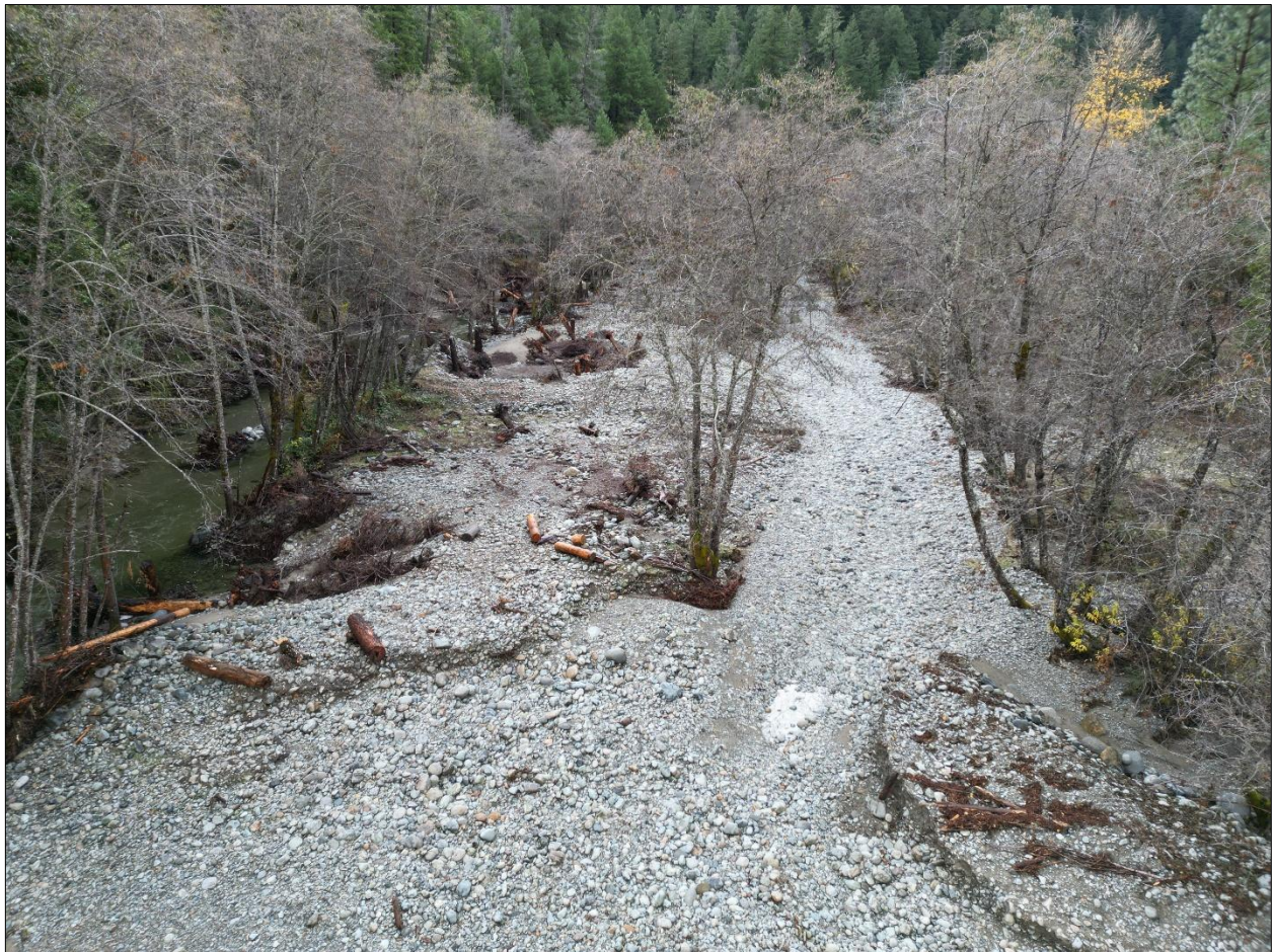
Image 52 (above): The Secondary Side Channel inlet on stream right between high flows. Note the scour through the constructed berm. November 26, 2024.
