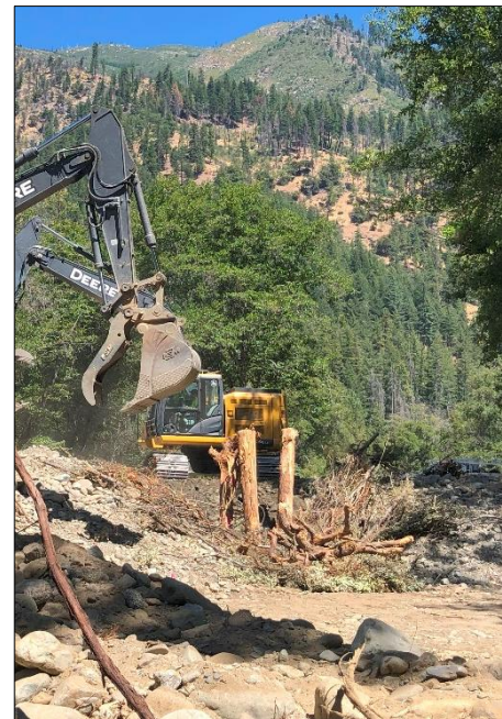
Image 42 (right): A Slot-EPA under construction. These features were constructed with logs, slash, cuttings, and fill material, and were then mulched.
