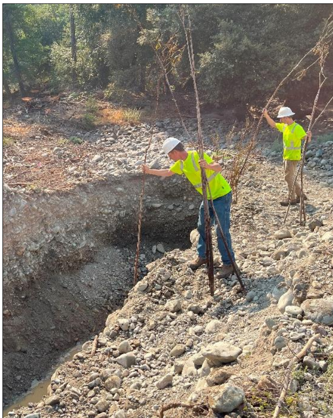
Image 43 (lower left): Contract crews placing live willow stakes into the baffles. Note the groundwater at the base of the excavated pit.
