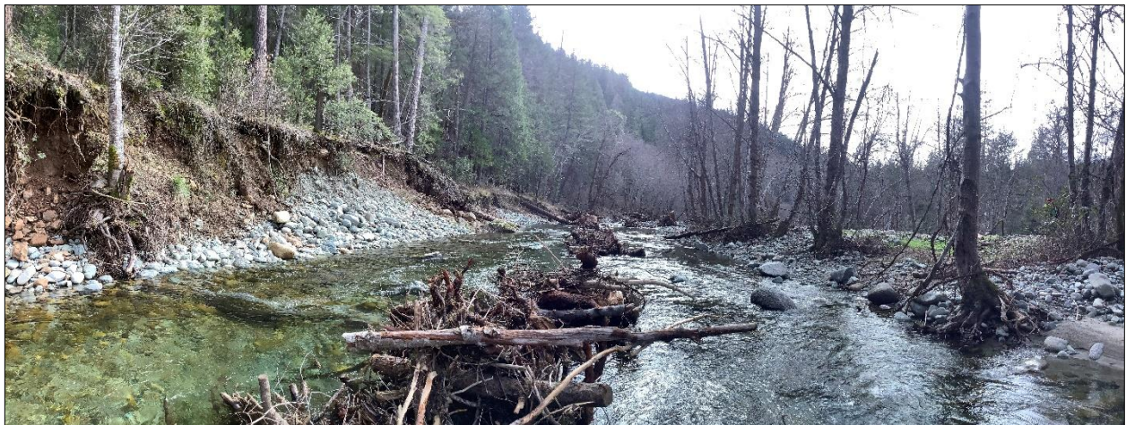
Image 22 (above): Post-phase one Perennial Channel Log Structures (facing downstream). March 2024.
