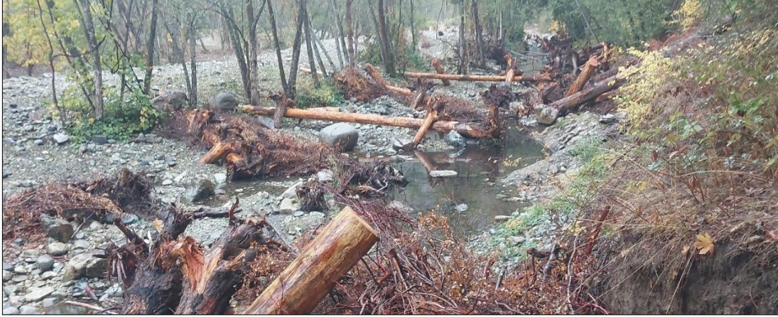
Image 25 (above): Perennial Channel Log Structures (facing upstream). November 1 st 2024
