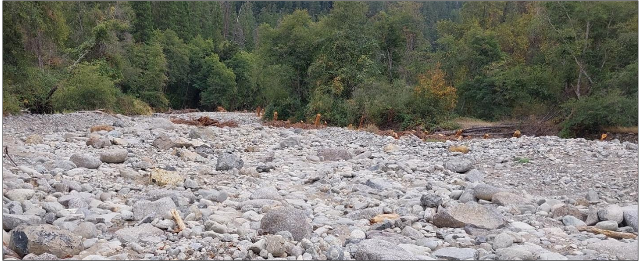
Image 53 (above): The Primary Side Channel log revetment completed in phase two of construction (seen center right). October 2024.
