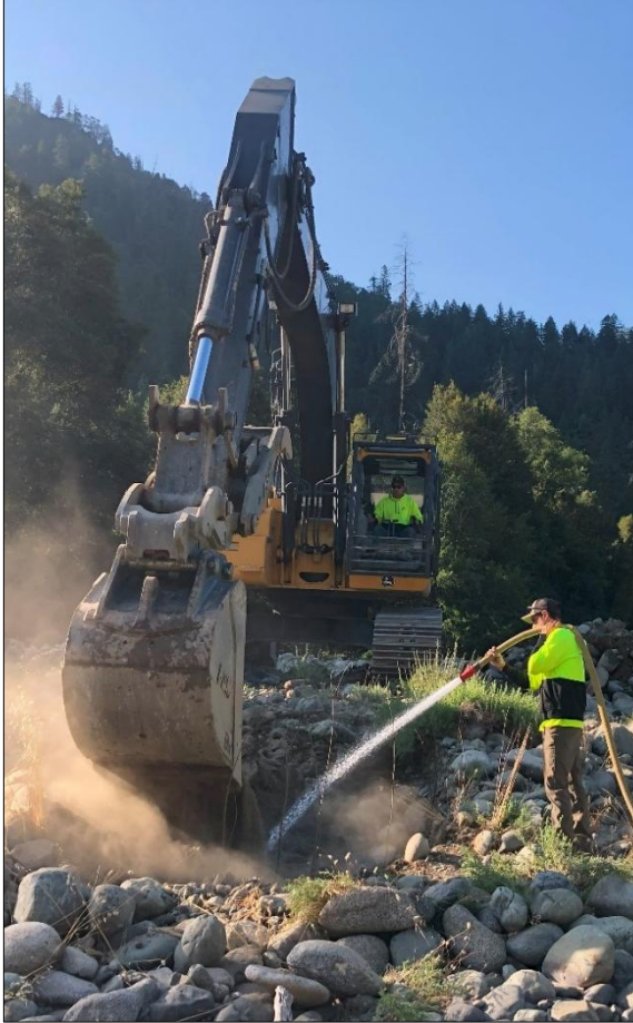
Image 44 (right): Contractors jetting fines into a willow cluster feature.
