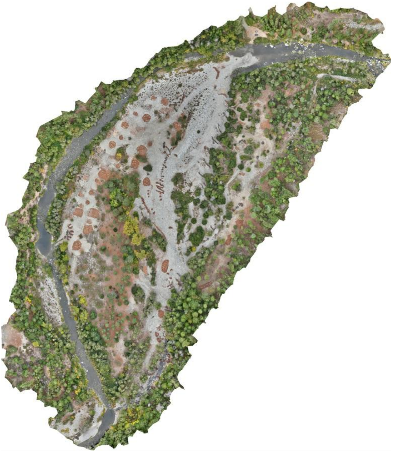
Image 3: Aerial of the project area post-phase two of implementation, October 2024. Credit: Mike Love & Associates (MLA). See the Interim and Final As-Built Plans for construction details. A final project map is forthcoming.
